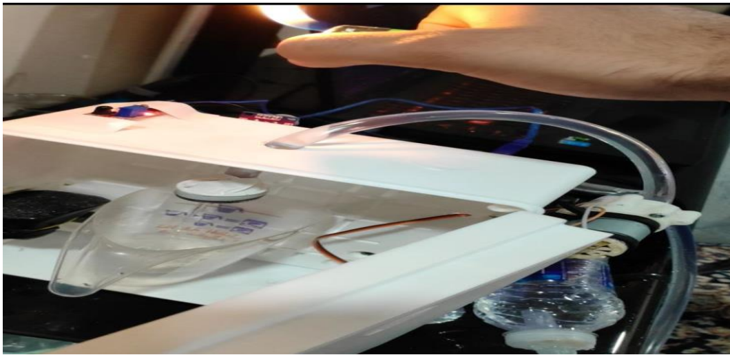
Fig. 6. Operates Water Pump When Detecting Fire.
