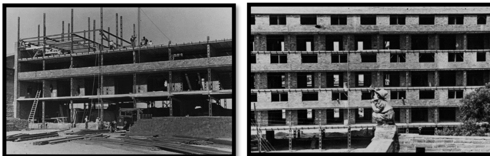
Fig. 3. A-B shows, the construction of the project, https://www.arquitecturacatalana.cat/en/works/casa-bloc
