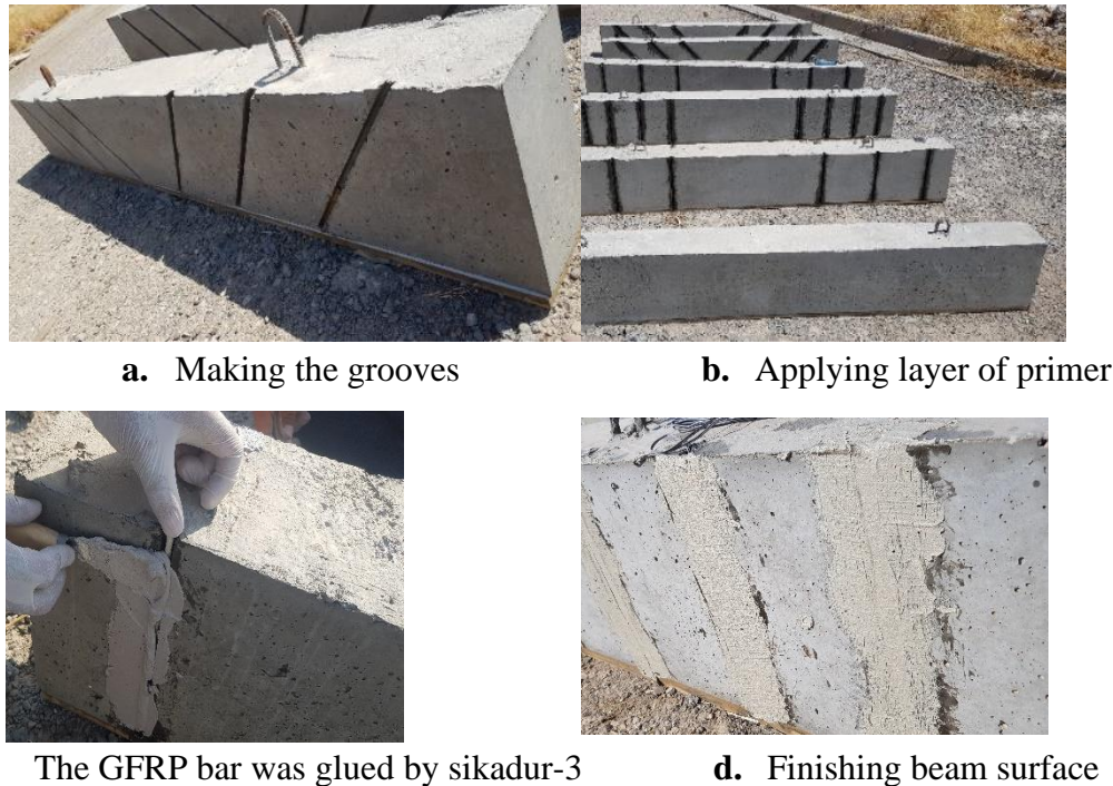
Fig. 2. Stages of installing GFRP bars
