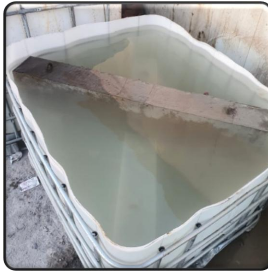
Fig. 9. Preparation details for casting the RC beams.
